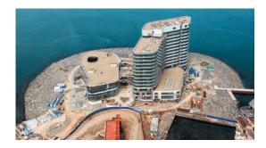
The configuration, location and number of floors of each detached building are dictated by the configuration of the plot and the preservation of a favorable insolation mode. Two buildings of the complex connected by a joint podium and by a glass junction.
